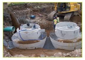
Even though the city of Fredericton has stormwater regulations in place requiring both quantity and quality control, this was an important site to have a Stormceptor, since all the stormwater from this site ends up in these sensitive wetlands. Thus, it is extremely important to keep hydrocarbons, Total Suspended Solids (TSS) and other pollutants out of New Brunswick waterways.
